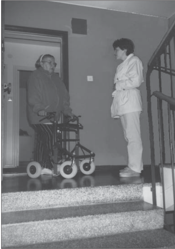
This building has no lift; the assistance of a home helper is needed to run errands. A lift would make independent mobility possible.
